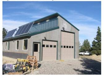
This picture is our barn as of spring 2015. Our rig is parked inside of there for the winter. It is NOT a house and it is fireproofed with the first coat of stucco. All exterior trim is made of cement board. Funny, I just noticed the power cord coiled up on the driveway that I run over to the tractor when I need to plug her in and heat the diesel up so she will start. Wait, I can do that without a generator or a power line? You bet I can!
