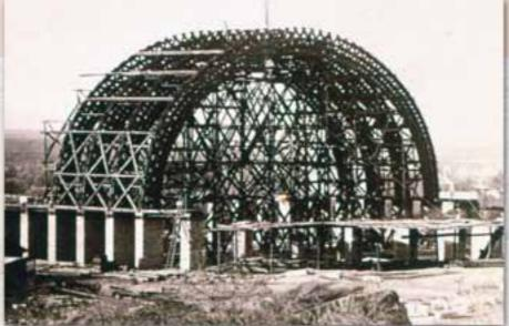
Above: The trusses were framed and put together on the ground and temporarily pinned. When everything was properly fitted and marked, the timbers were taken apart and raised plank by plank and put into place over scaffolding erected for that purpose.
