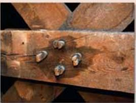
Above: Detail showing the orientation of the wedges. The wedge, driven into the peg, expanded the peg to ensure a tight fit. The wedge was driven so that it expanded in the direction of the grain to avoid splitting the trusses at the end. Contrary to legend, some metal bolts were used in the construction of the Tabernacle.
